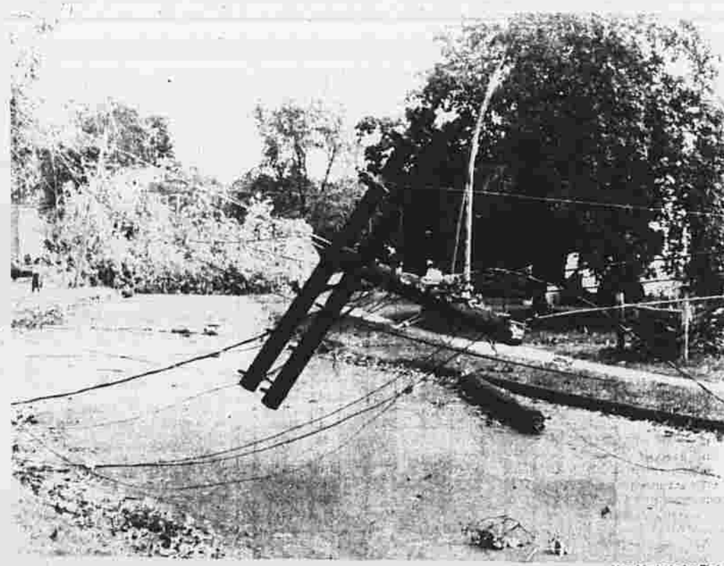
A utility pole on Crestwood Drive could not withstand Gloria's winds Friday as it split into three pieces, spreading its wires from one end of the street to the other.
