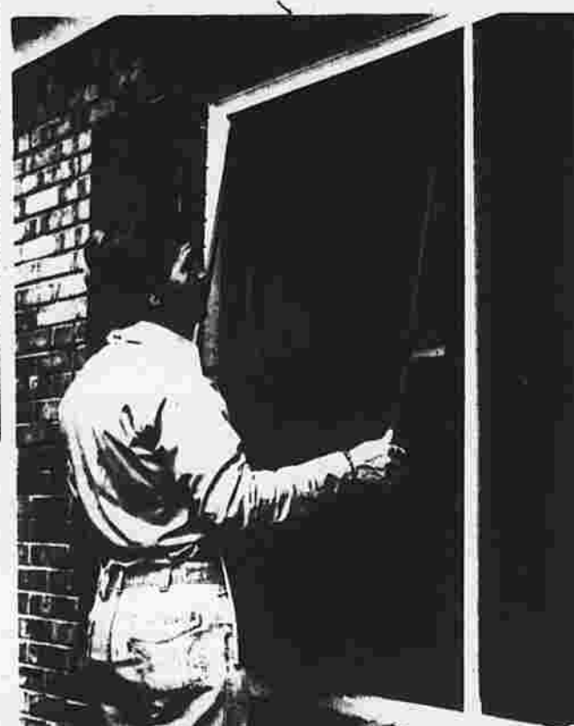
Solar screens can make even storm windows more energy efficient and help reduce fading and glare year-round. They can be installed on any type or size of window.
